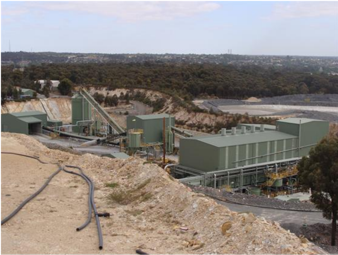
Figure 1 – Unity Gold Plant at Kangaroo Flat looking north towards Bendigo
